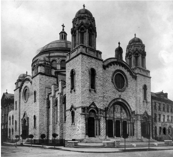
Historic Exterior Photograph
