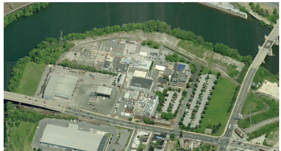
PENN'S SOUTH BANK - AERIAL VIEW OF THE EXISTING CONDITIONS
