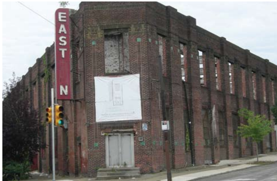
The former Eastern factory at 30th Street and Cecil B. Moore Avenue that SMCDC and SMNAC are working on getting redeveloped.
