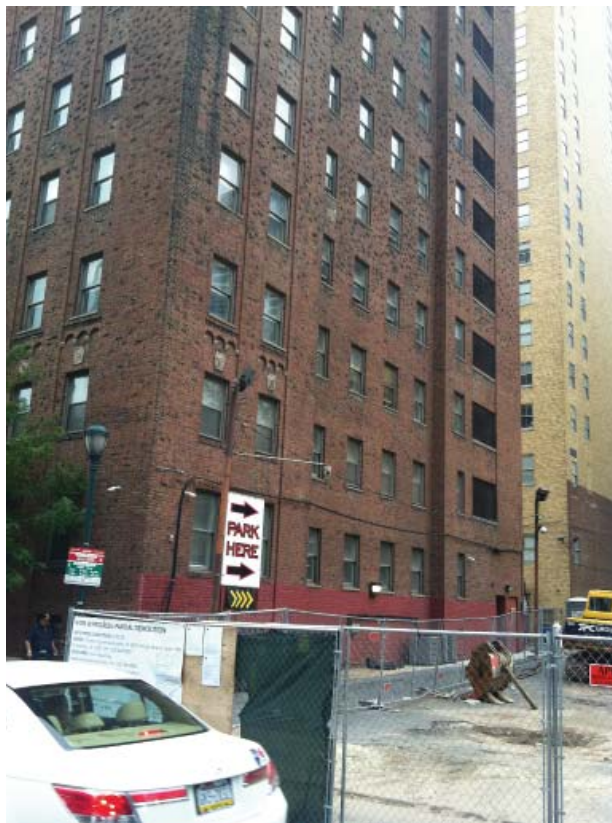
5 east facade of kate's place from sansom
