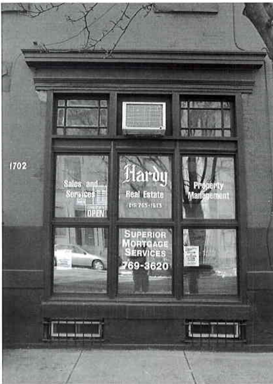
Thin wood muntins and decorative cornices are typical storefront details.
