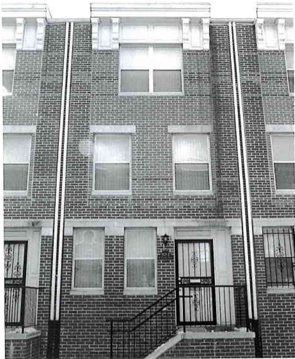
These contemporary houses follow the cornice line and materials of older, neighboring houses, yet announce their 20th century construction.
