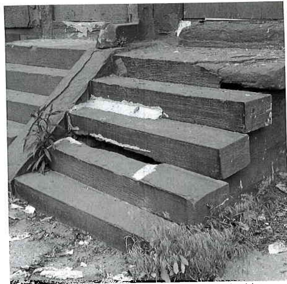
Masonry steps should be maintained to prevent the damaging effects of water penetration and subsequent freezing and thawing, as seen on the right.
