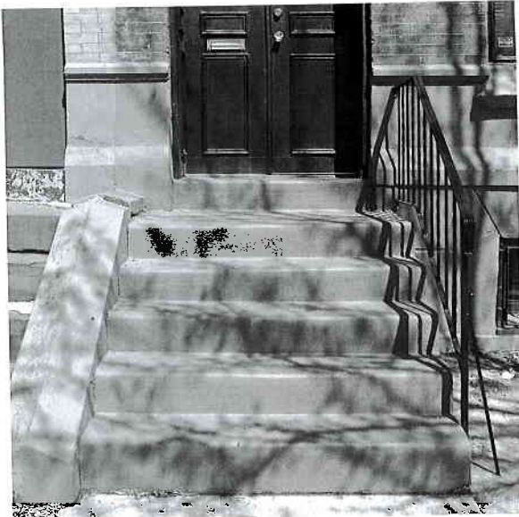
Masonry steps should be maintained to prevent the damaging effects of water penetration and subsequent freezing and thawing, as seen on the right.
