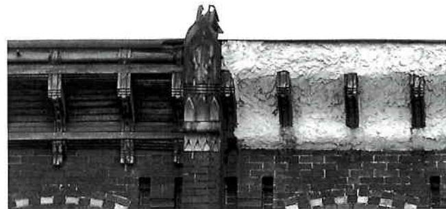
Stucco and aluminum cladding hide architectural details.
