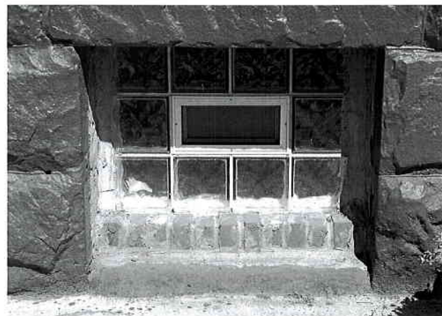
Glass block should not be used to replace a basement window.
