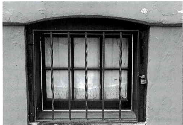
Original basement window.
