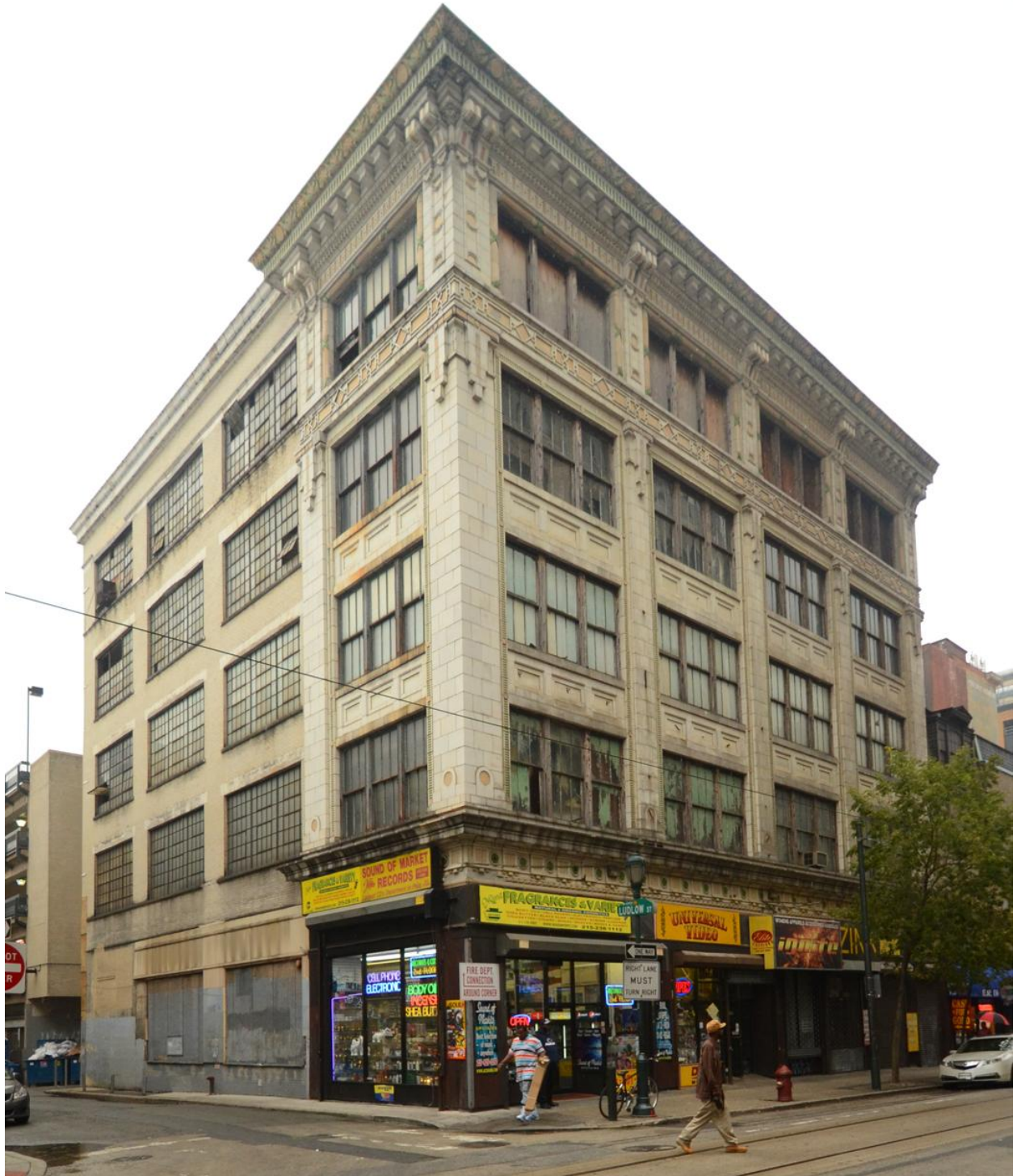
Figure 1: North (left) and west (right) elevations as viewed looking southeast.
