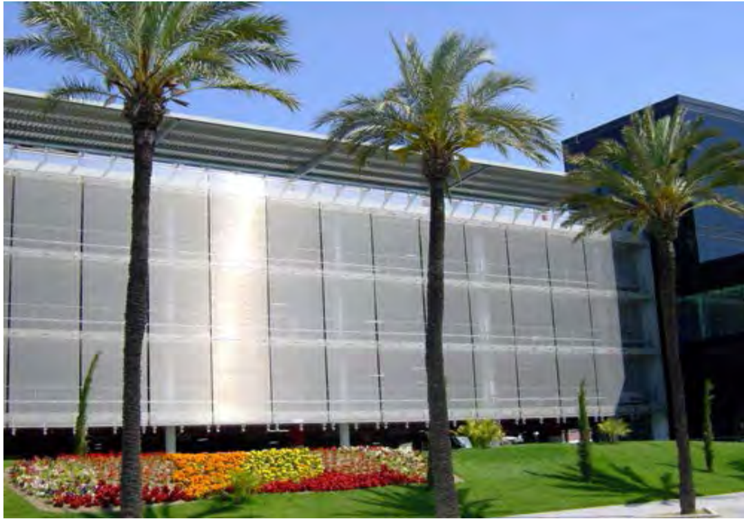
PERFORATED METAL DURING THE DAY
