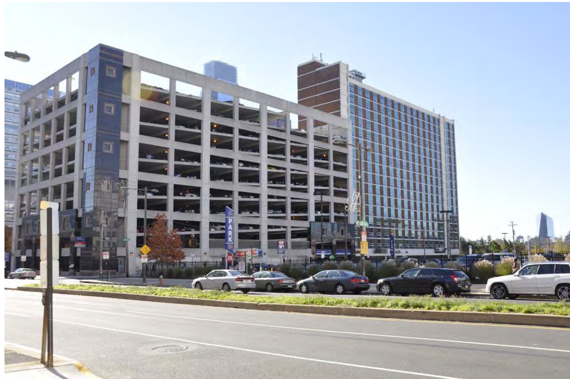
1 | VIEW FROM NORTH BROAD LOOKING SOUTHWEST
