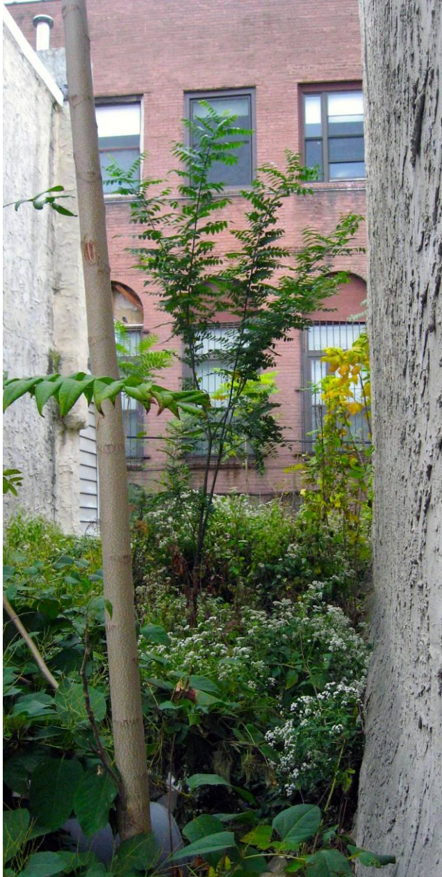
Figure 6K: Fenestration pattern along the Stiffel Center's east elevation. Photo taken from 2506 South 6 th Street, looking west, through the an opening in the fence that currently fronts a vacant lot.
