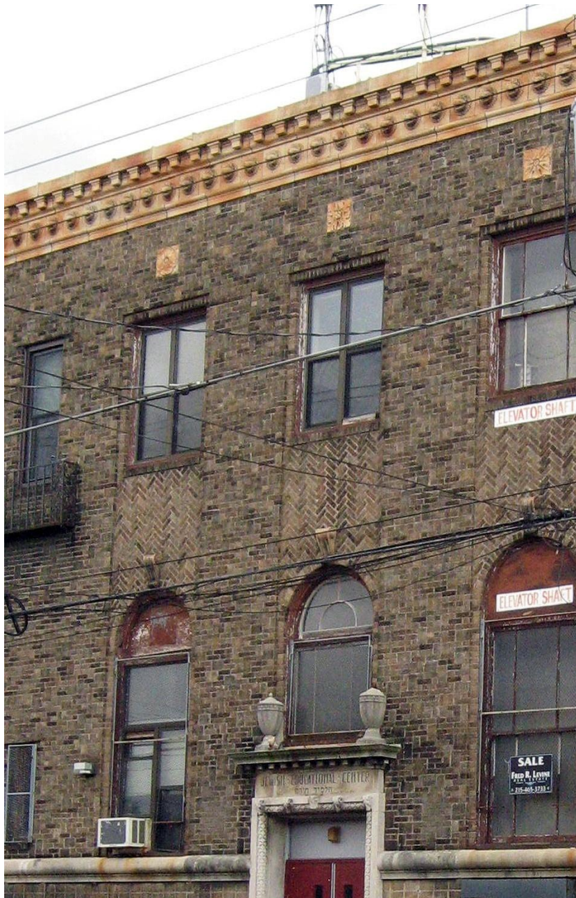
Figure 6F: North-facing, Porter Street façade detail showing the two above-basement-level stories, the balconette, cornice, keystone, and brickwork detail.
