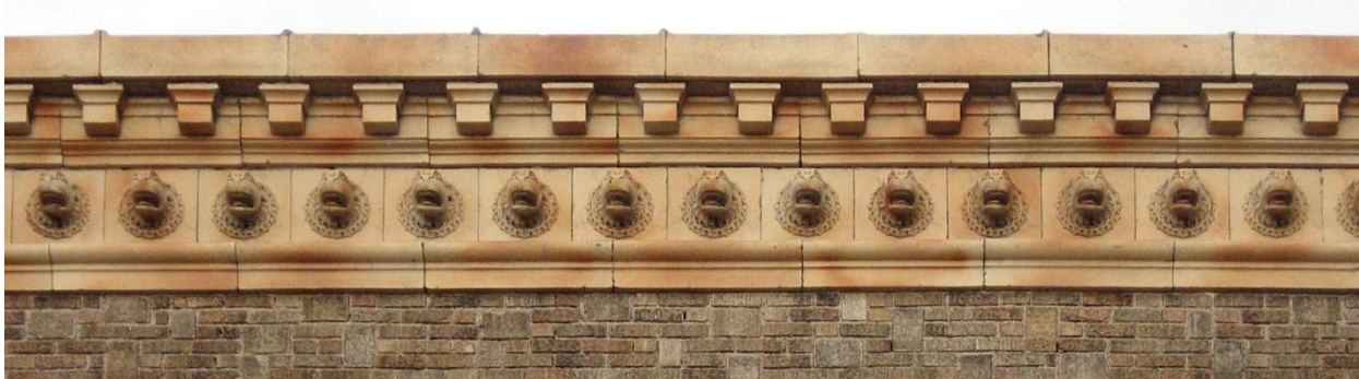
Figure 6G: Detail of cornice
