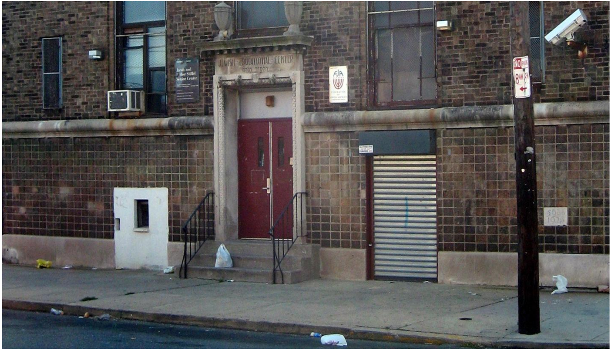
Figure 6C: Base of the north elevation
