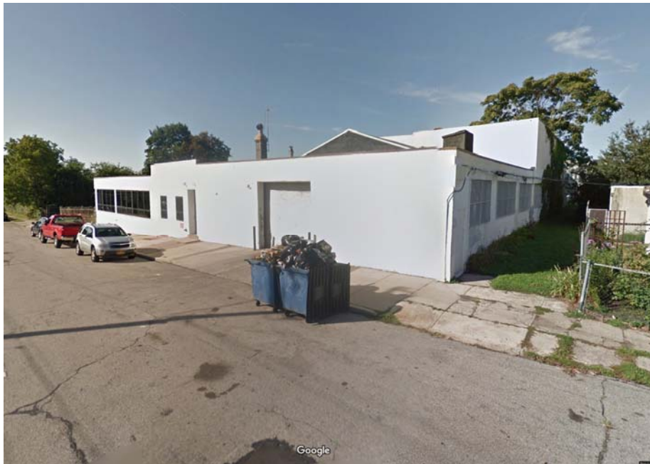
Photo 2 – looking south at existing garage on site
