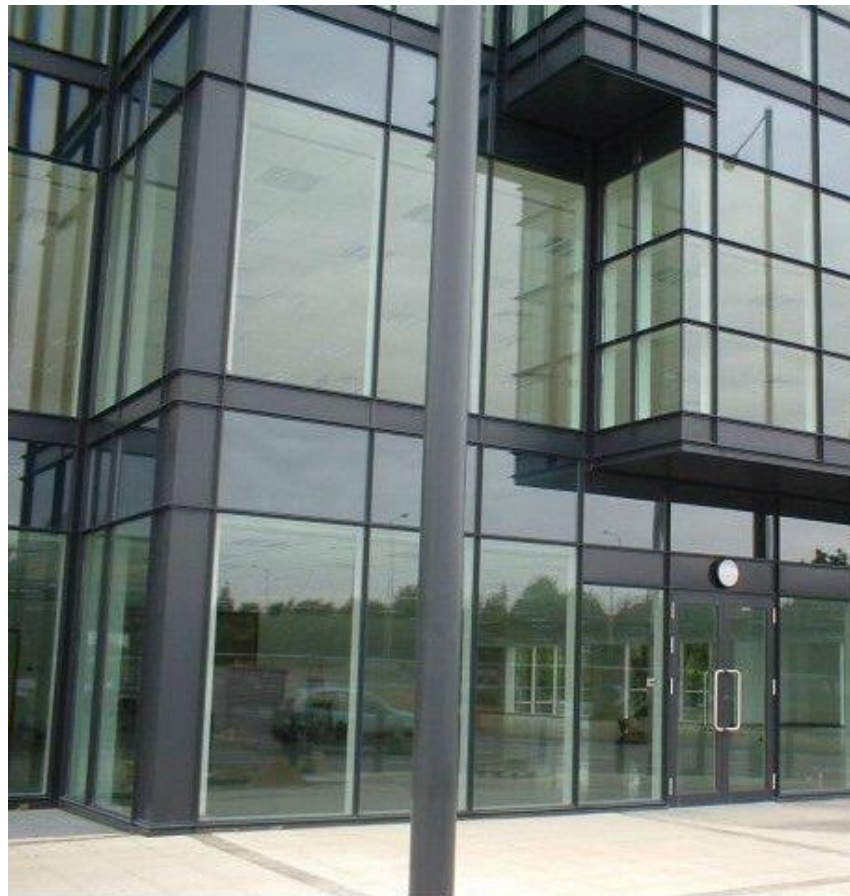
Black curtain wall grids w/ clear & blue green spandrel glass
